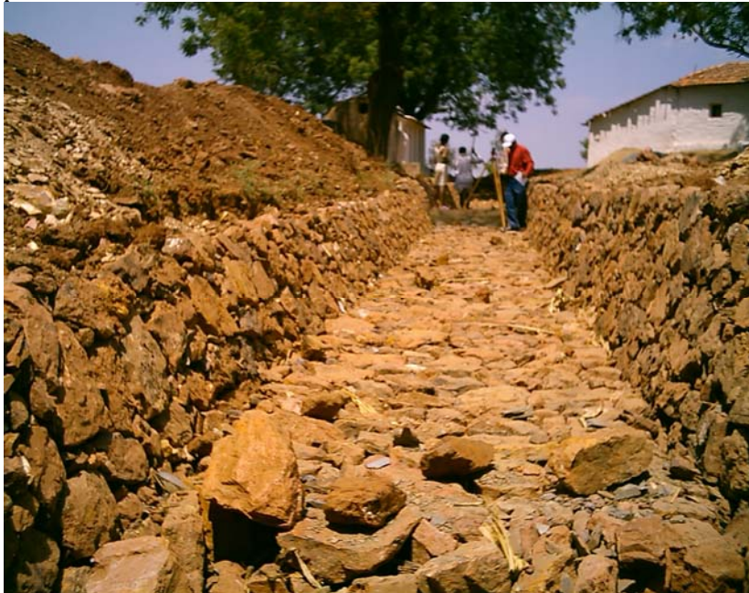
Feeder Channel is under construction.
