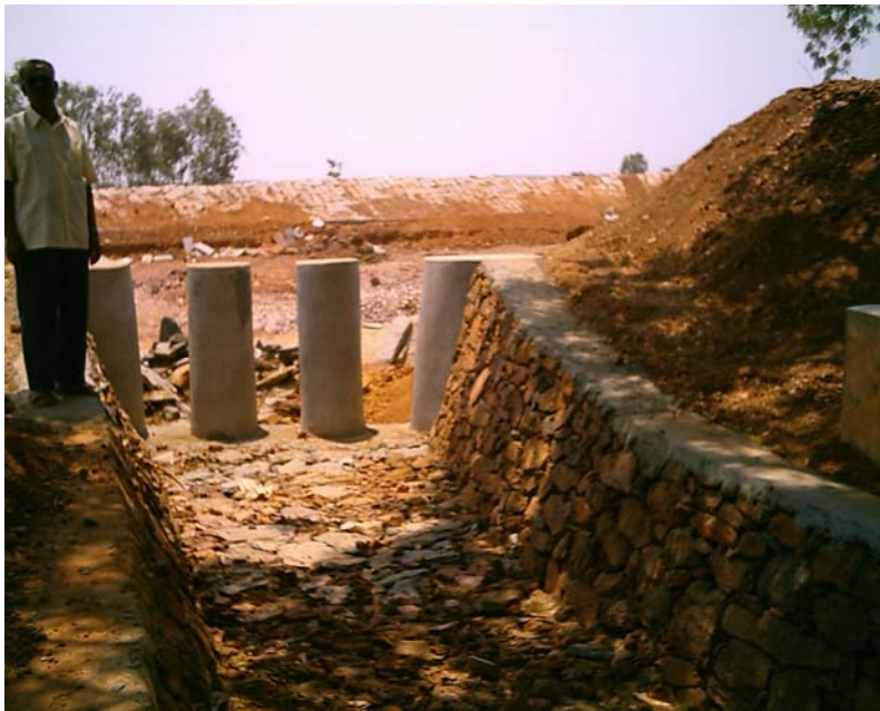
Tank rehabilitation work under progress.
