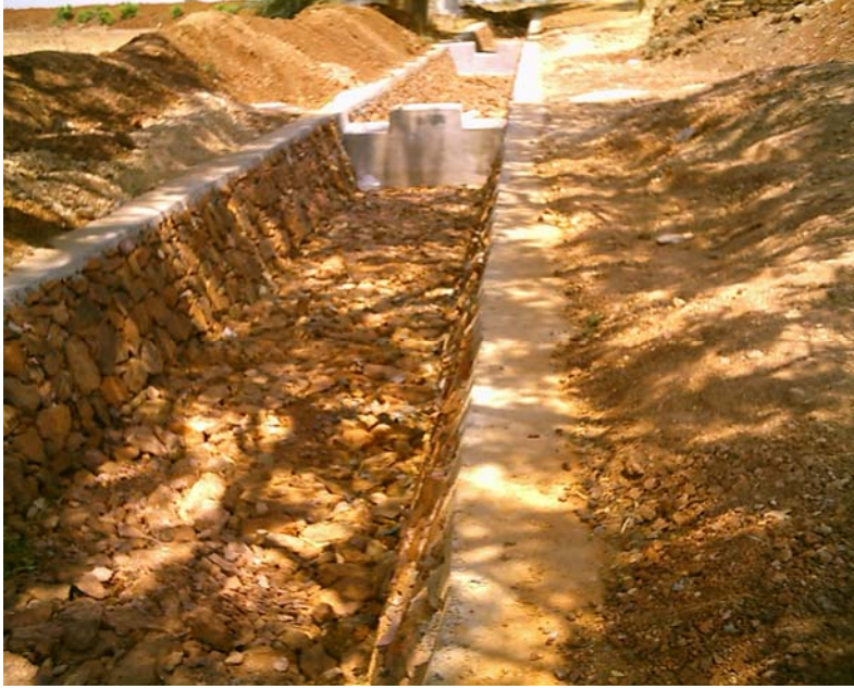
Feeder channel under construction
