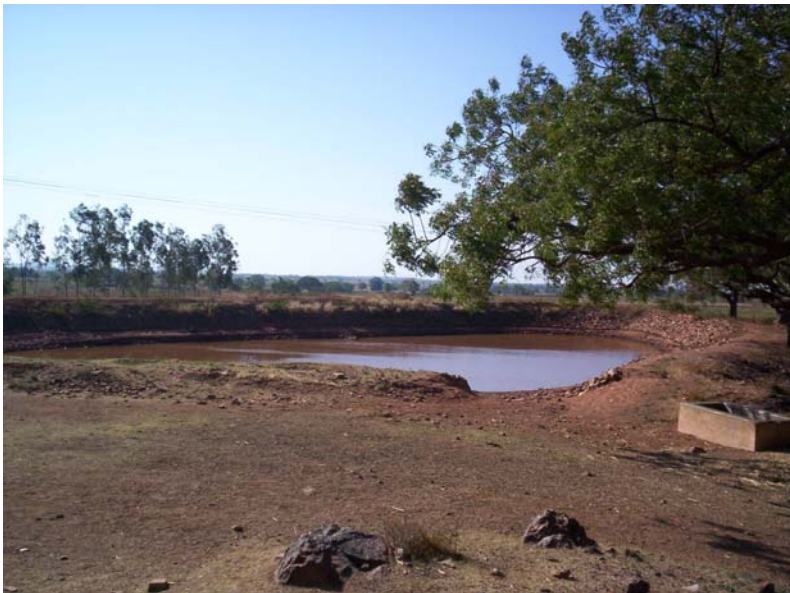
Tank before rehabilitation
